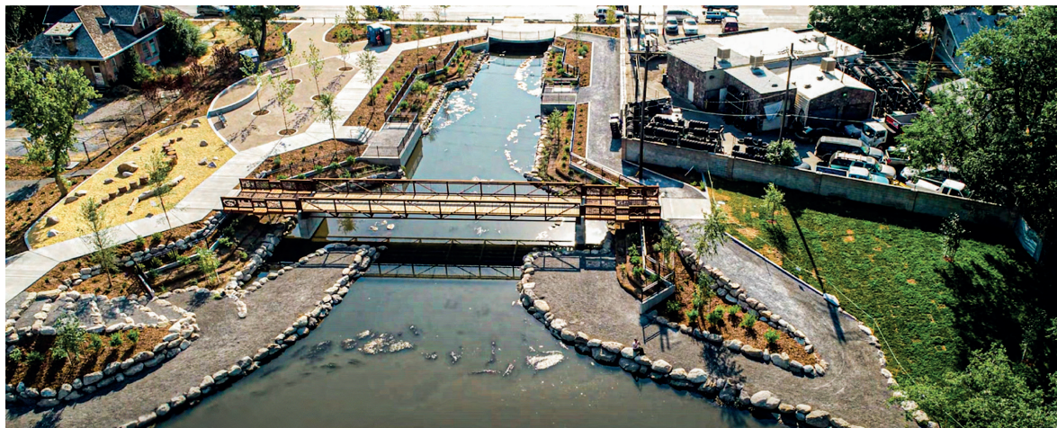
Over $3 million was secured to uncover 200 feet of combined stream in a newly restored channel, construct a 120-foot bridge to connect the site to the Jordan River Trail, and add a public plaza.
