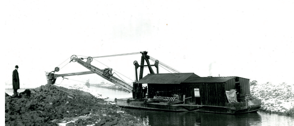
Dredging the Surplus Canal on the Jordan River, June 1913. Used with permission, Utah State Historical Society.
