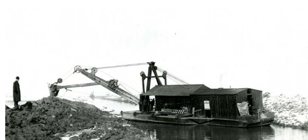
Dredging the Surplus Canal on the Jordan River, June 1913. Used with permission, Utah State Historical Society.
