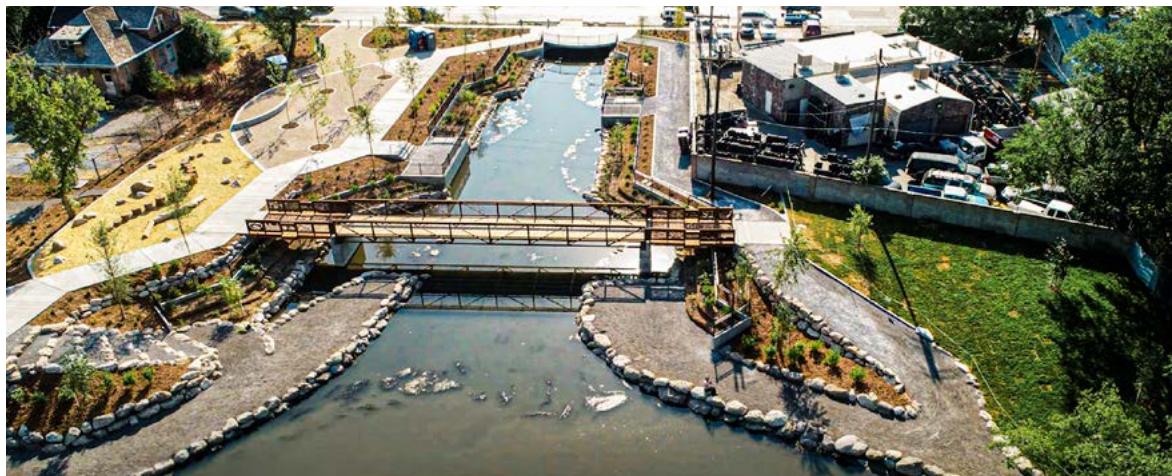
Over $3 million was secured to uncover 200 feet of combined stream in a newly restored channel, construct a 120-foot bridge to connect the site to the Jordan River Trail, and add a public plaza.
