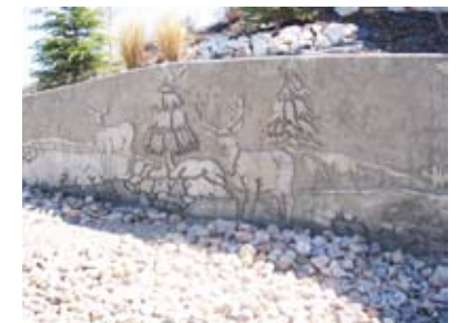
ALONG THE JORDAN RIVER PARKWAY, A RETAINING WALL AND HIGHWAY OVERPASS HAS BEEN TURNED INTO PUBLIC ART
