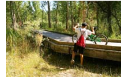
BICYCLISTS HAVE DIFFICULTY ACCESSING SOME TRAIL SEGMENTS
