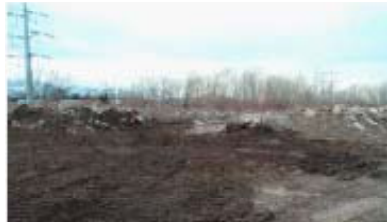
DURING DEBRIS REMOVAL
