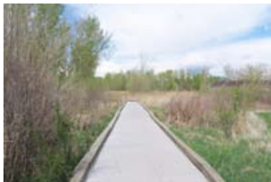
ELEVATED WALKWAYS ENABLE PEOPLE TO ENJOY THE RIVER AREA WHILE PRESERVING WETLANDS FOR NATURAL STORMWATER FILTRATION
